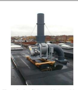
Figure 2 – Roof Mounted Exhaust Blower
