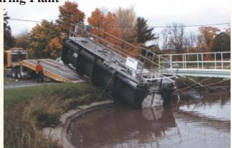
The three million gallon lagoon has two five horsepower splashers operating during the Department of Environmental Conservation (DEC) Summer Permit discharge conditions from May to November. During the summer, the undiluted whey-waste water in the lagoon is drawn down and sprayed onto the adjacent meadow, which is owned by the cheese manufacturer.
